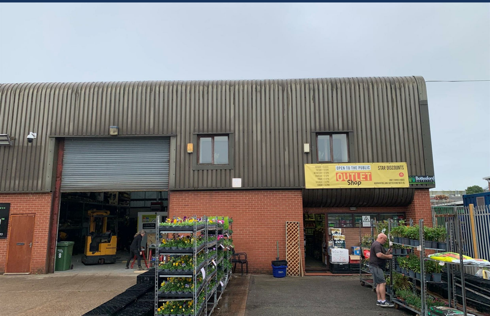
First floor office 1, Ranch House, Normanton Lane, Bottesford NG13 0EL
